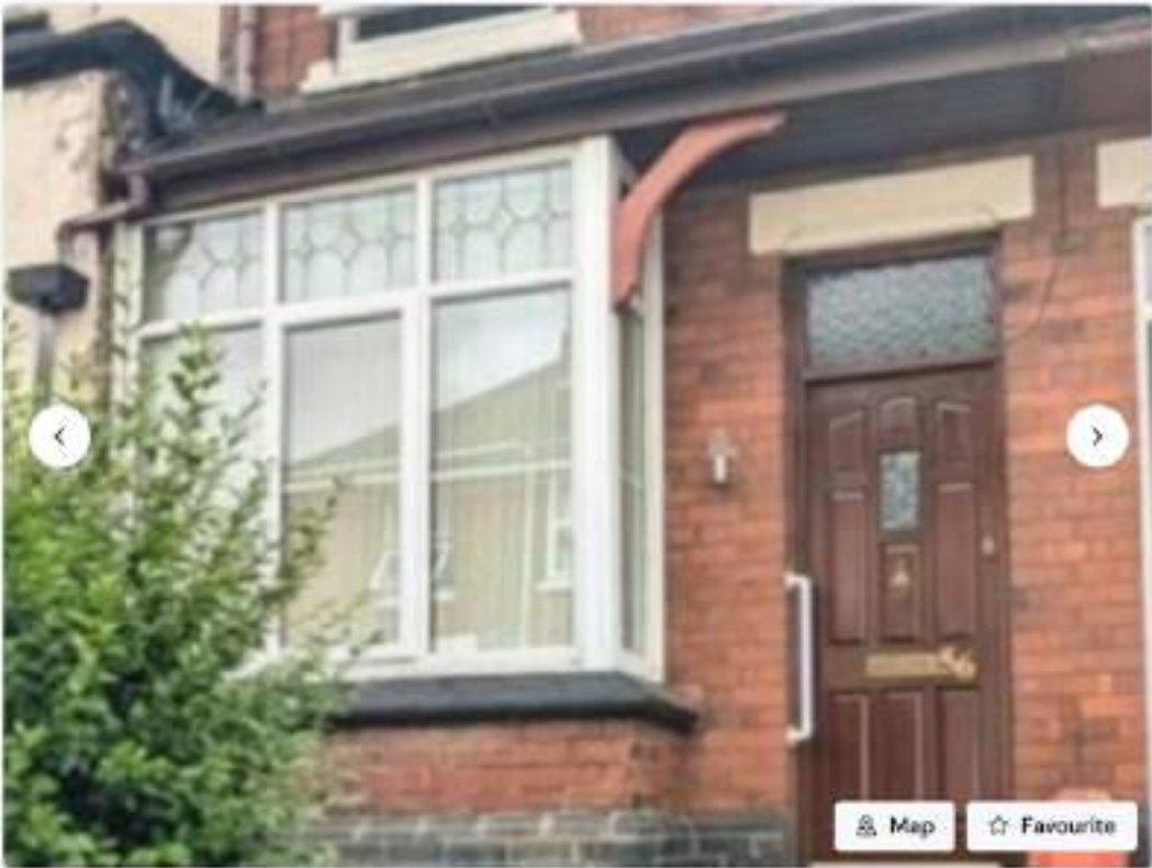
2 Bed Terraced House, Cromartie St, ST3
