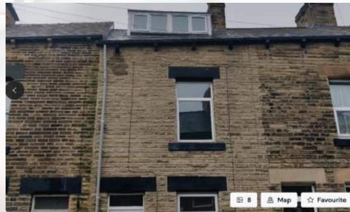
2 Bed Terraced House, Wharnccliffe Street, S70
